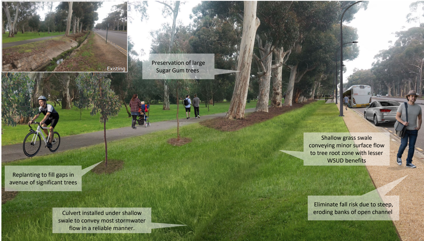
Rehabilitated drainage channel looking north-west along Glen Osmond Road and Ponder Avenue
